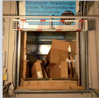
Feed opening through wall
