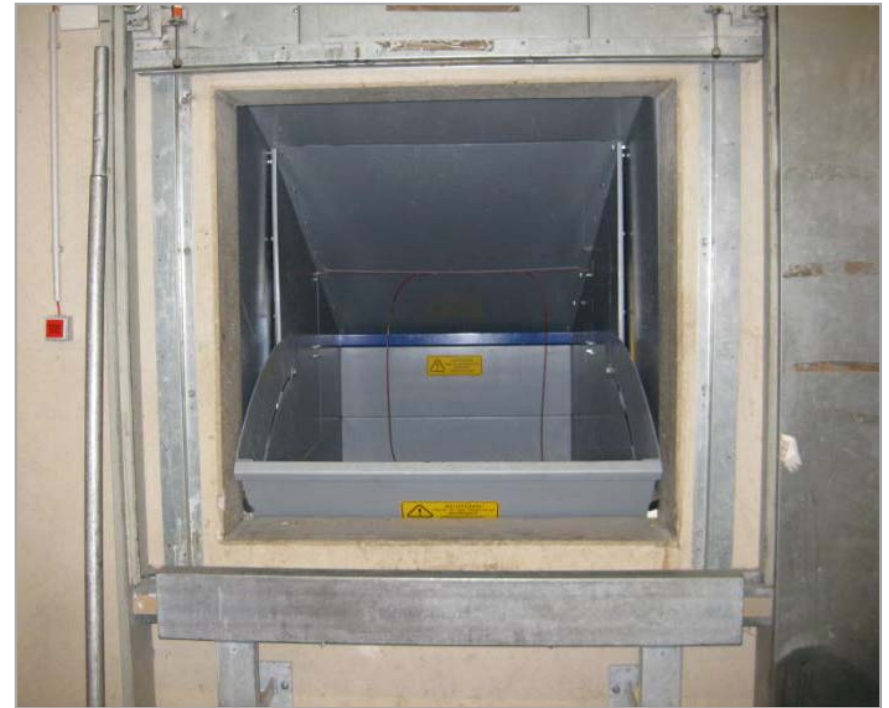
Feeding from inside through a wall mounting
